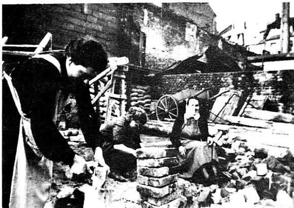
Cleaning the old bricks from our bombed church in Frankfurt to build the new building (1953).
